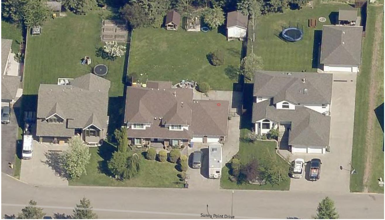
Image.3 Currently, the single-detached dwelling on the parcel has a double garage. When not in use, the owner parks the RV on the paved driveway next to the house. Widening the driveway to 10 m as proposed will allow the owners to safely park the RV, without causing any damage to the house.
