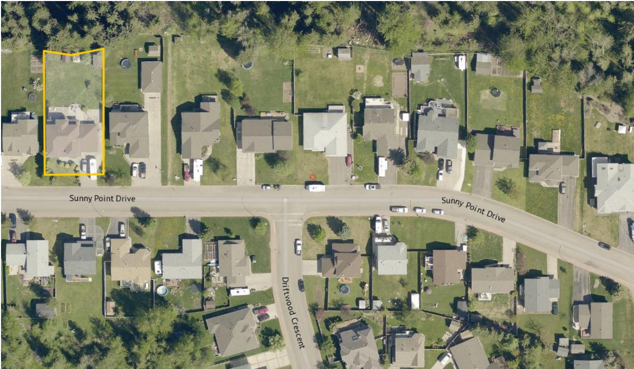
Image 2: The property, which has a 24 m street frontage, is accessed off a 7-m driveway from the fronting street; the Applicant’s proposal is to widen the driveway to 10 m in order to ensure safe RV parking on the side yard.
