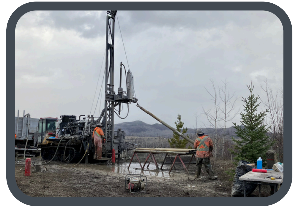
Airport Geotechnical Drilling
