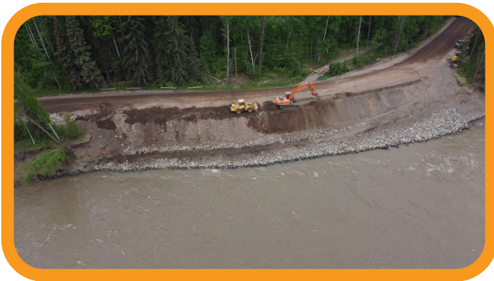
Emergency Bulkley River Bank Armoring
