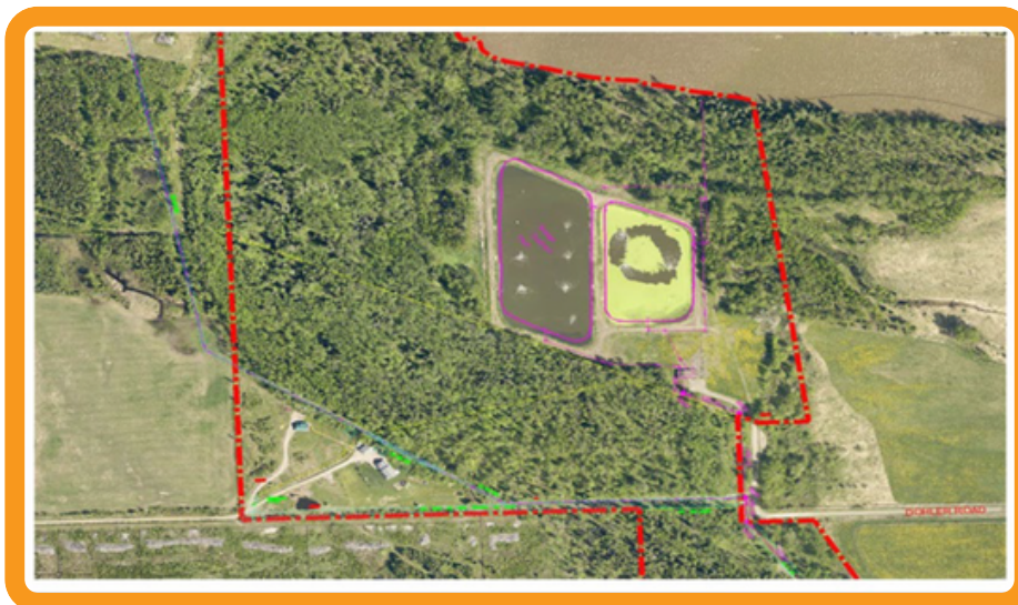
Aerial view of the Wastewater Treatment Plant
