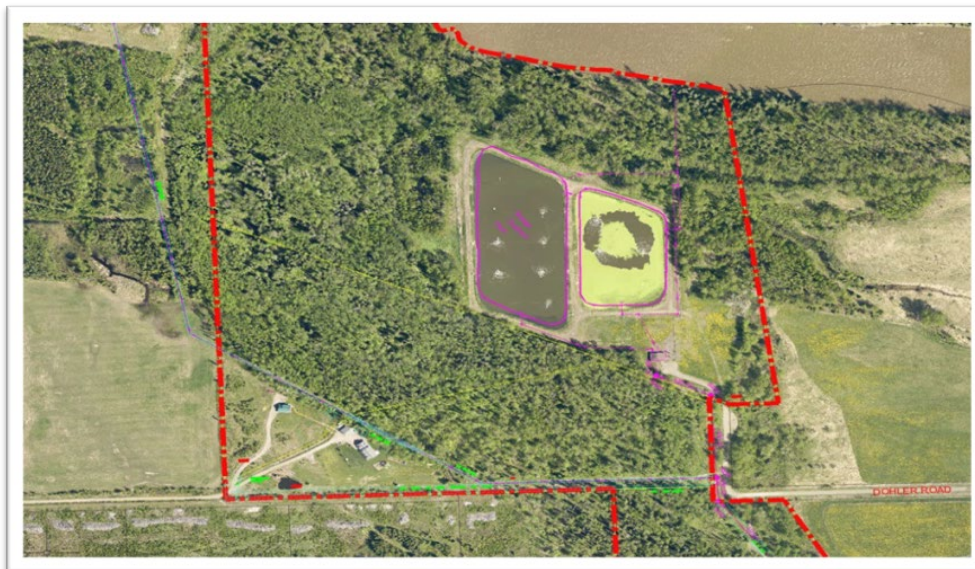
Aerial view of the Wastewater Treatment Plant (July 2021)
