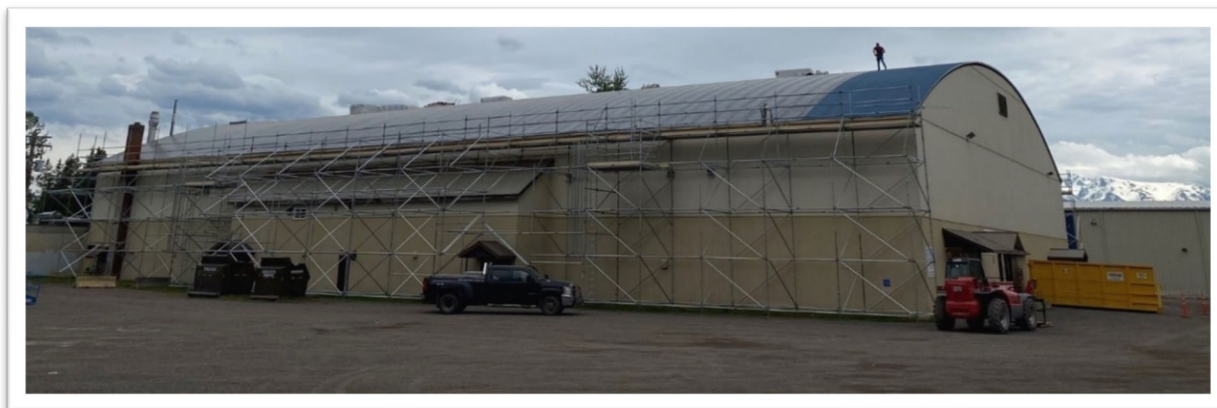
Civic Centre Re-roofing Project
