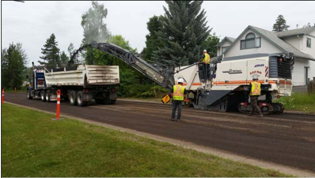
Milling Machine Removing Old Asphalt in Preparation for New Asphalt Paving
