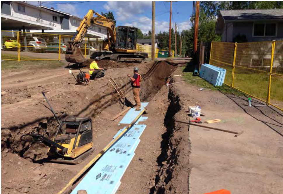
Photo (above): 14th Avenue water main replacement project
