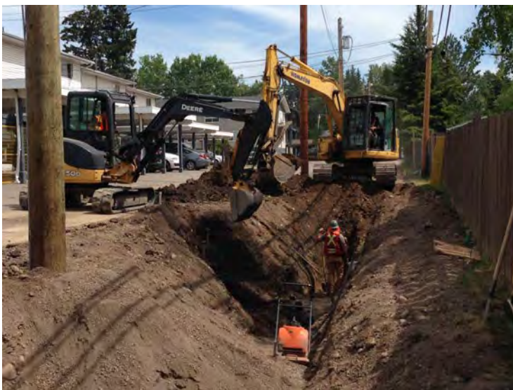
Photo (above): 14th Avenue water main replacement project, June 2018.
