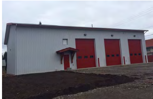
Photo (above): Fire Training Centre March 2019
