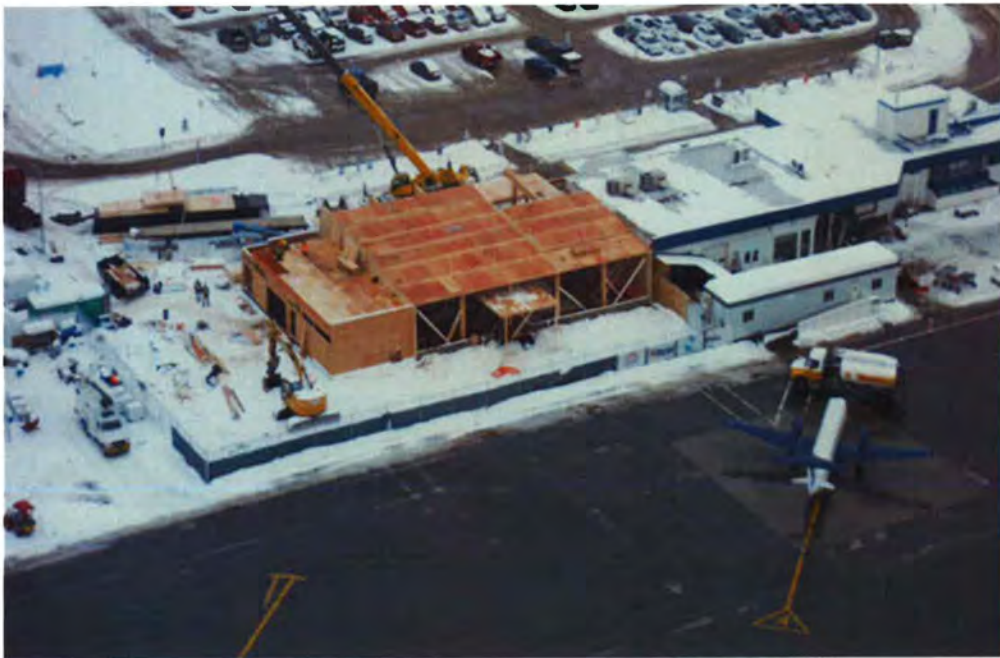
Airport Terminal Construction as of December 2017
