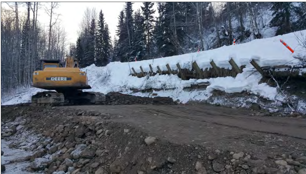
Photo (above): Rosenthal Road repair.
