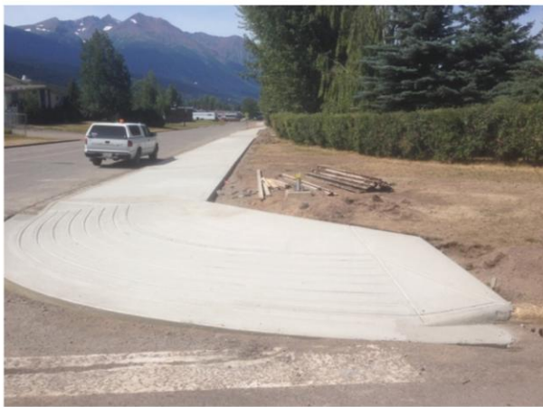
Above 3 Photos: New Fulton Avenue Walkway.
