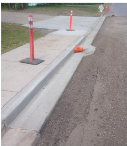
Photo: New Lane and Curb along 16 th Avenue.
