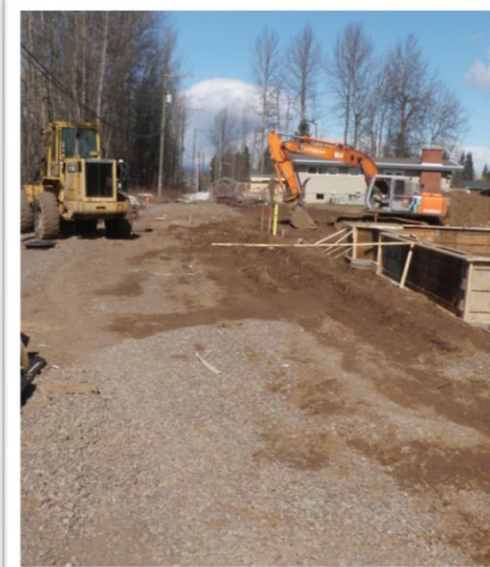
Photo: New "Four-Plex" development along Third Avenue and Vancouver Street.
