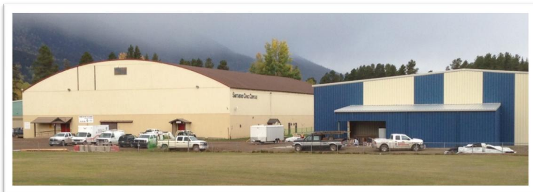
Photo: October 1, 2014 – Construction of the New Smithers Arena.
