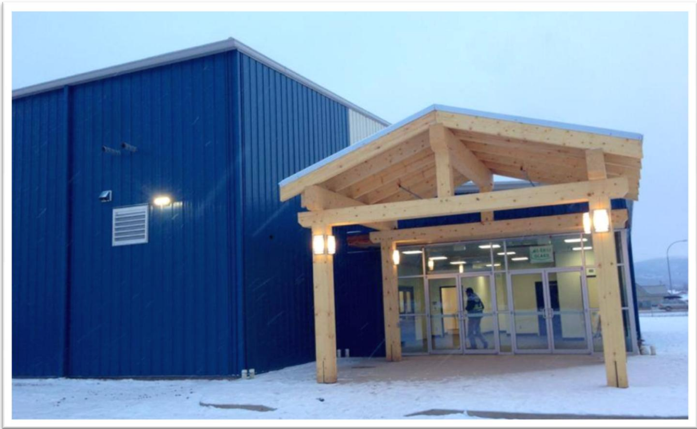
Photo: New Arena reaches “Substantial Completion” December 2, 2014.
