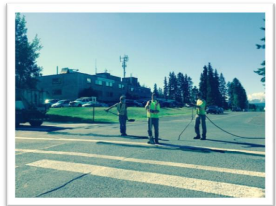
Photo: Crews crack sealing a road
