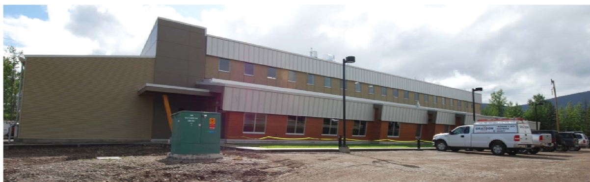
INDUSTRIAL WINNER: 2715 Tatlow Road (Hy-Tech Drilling)
