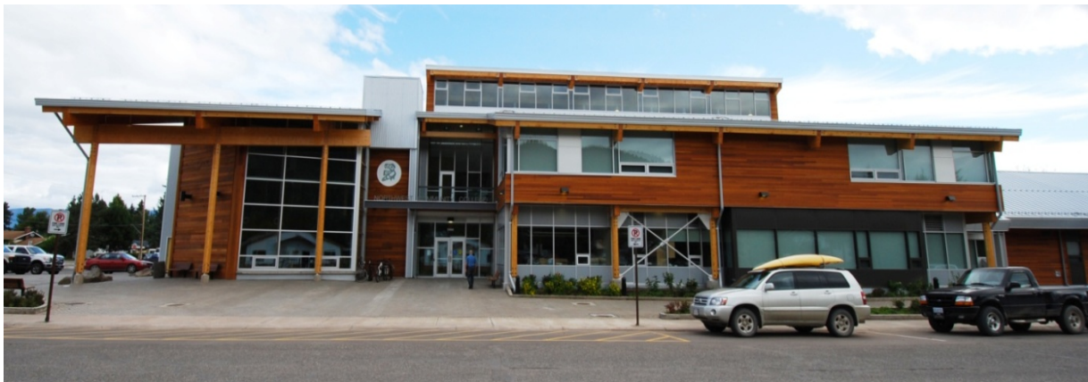
NORTH WEST COMMUNITY COLLEGE EXPANSION: 2ND AVENUE
